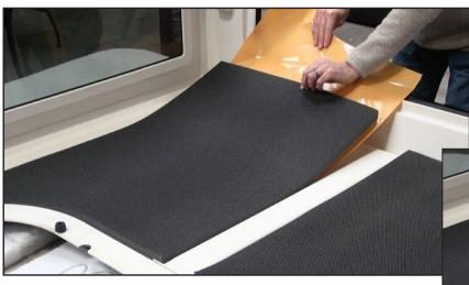
FIG. 11 & Fig 12 Slowly pull the release liner off as you press the piece into place. NOTE: Use gentle pressure. DO NOT use a lot of pressure when pressing piece into place.
