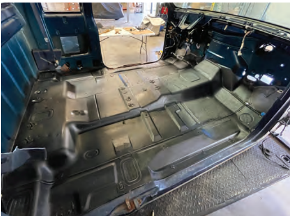
FIG. 1 Remove seats, console & carpet. Clean dirt/debris and recommend using sealer on any rust spots (View from passenger side)
