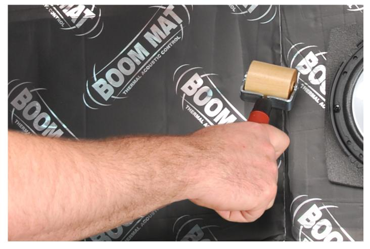
**USE INCLUDED INSTALLATION ROLLER TO PRESS DAMPING MATERIAL IN PLACE TO ENSURE GOOD ADHESION**
