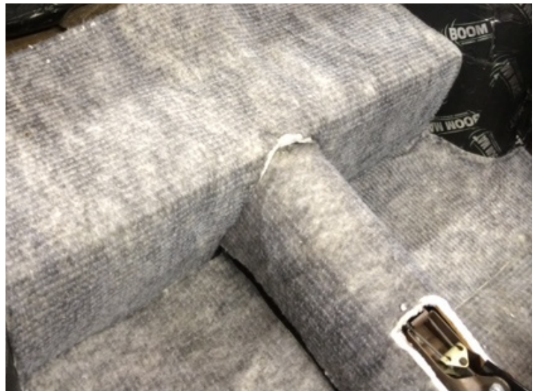
UC Lite installed with gray side up.
