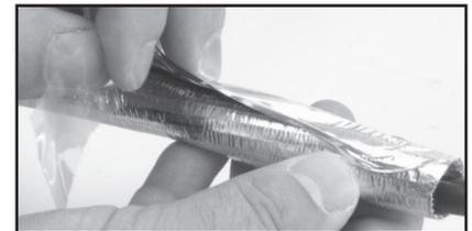
STEP 4. Slide the sleeve up the line as you go while pressing the flap closed until you cover that end of the line.
