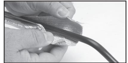
STEP 3. As you wrap the line, peel back the adhesive backing & fold over the adhesive flap pressing down to close the sleeve.
