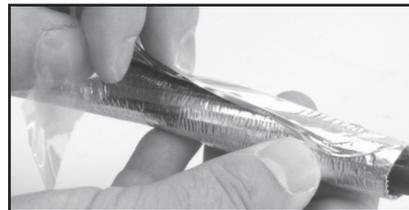
STEP 4. Slide the sleeve up the line as you go while pressing the flap closed until you cover that end of the line.
