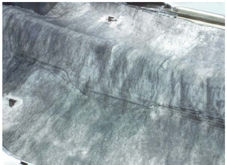
UC Lite installed with gray side up.
